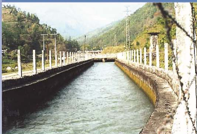
Open Power Canal, Sunkoshi HPP
