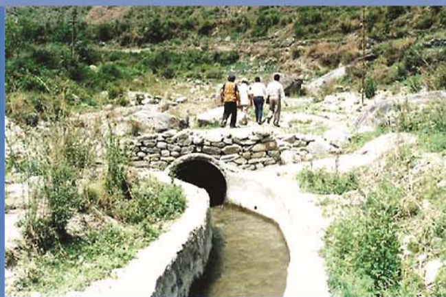
Closed Conduit and Open Canal, Chilime HPP
