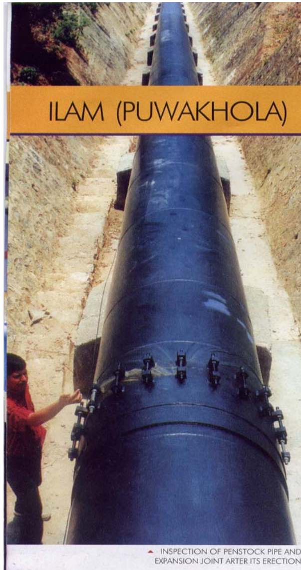
Figure 3.37: Penstock of Puwa Khola HPS showing Expansion Joint
