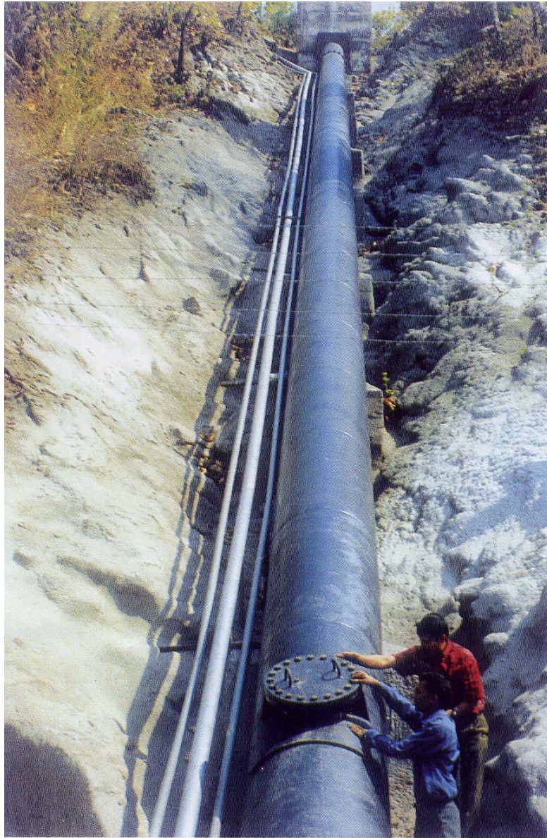
▲ INSPECTION OF PENSTOCK PIPE MANHOLE
