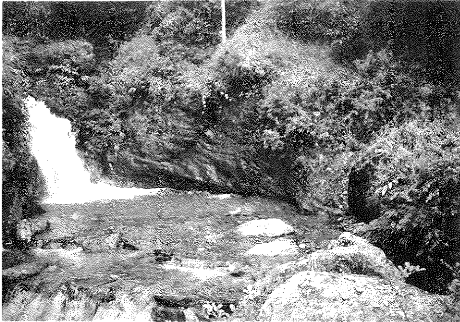
Photograph 1A Ideal Location for Simple Side Intakes
