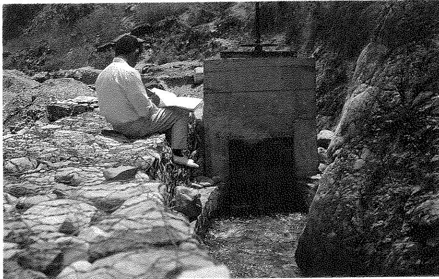
Photograph 1D Side Intake Built Behind Gabion Protection
