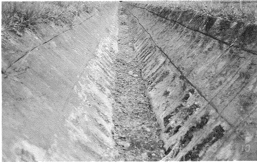
Photograph 7B A Brick-Lined Canal with a Trapezoidal Cross-Section
