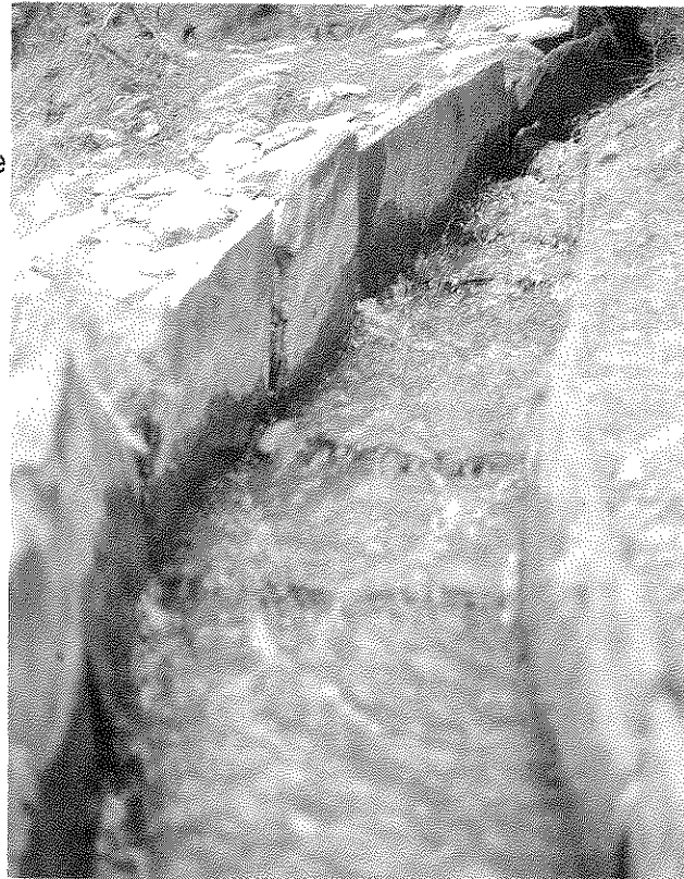
Photograph 7G A Slate-Lined Canal
