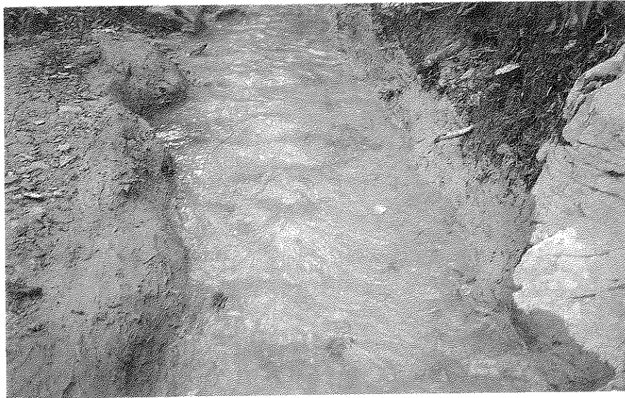
Photograph 7H Soil-Cement Lining has Effectively Controlled Seepage in this Canal
